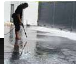
6 Wash the Surface
